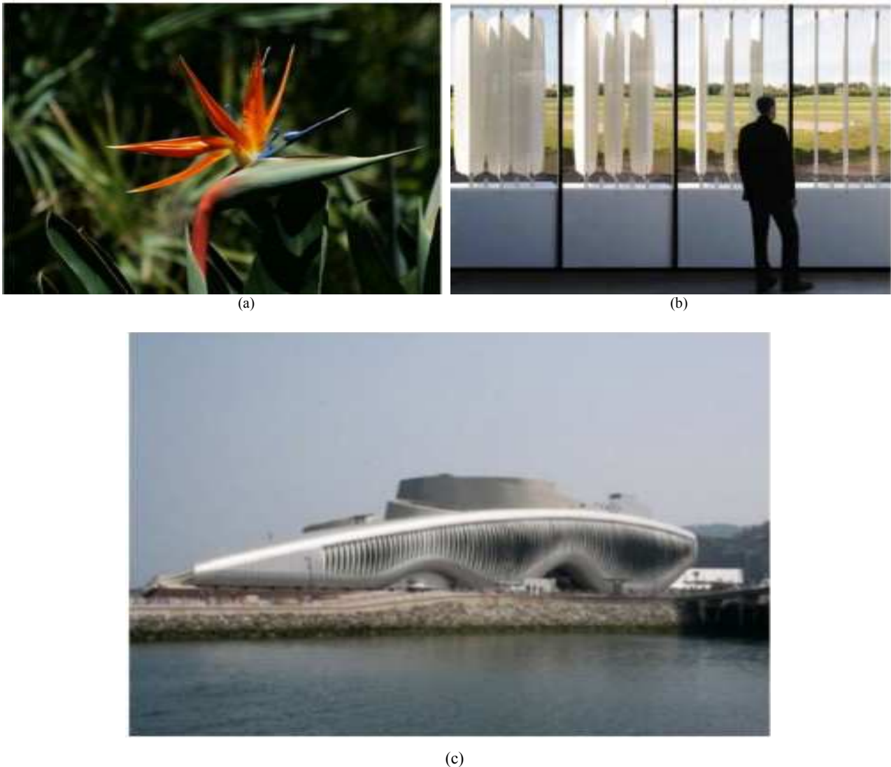
Fig. 7. Flectofin® shading systems for adaptive façades. (a) the Bird-of-Paradise flower (source: www.asknature.com ) (b) full scale prototype for the Flectofin® principle (picture taken from (Lienhard et al. , 2011)); (c) the Theme Pavilion for Expo 2012 in Yesou, South Korea, by Soma Architecture (source: www.compositesandarchitecture.com )
