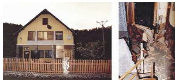
Fig. 2. External and internal view of the objects damaged by the flyrocks
