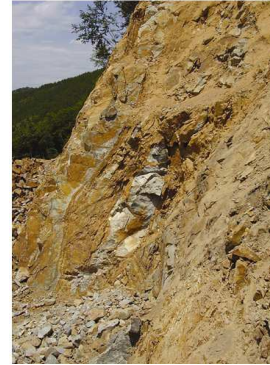
Fig. 6. The relic of fresh andesite in altered andesite mass at the bench slope
