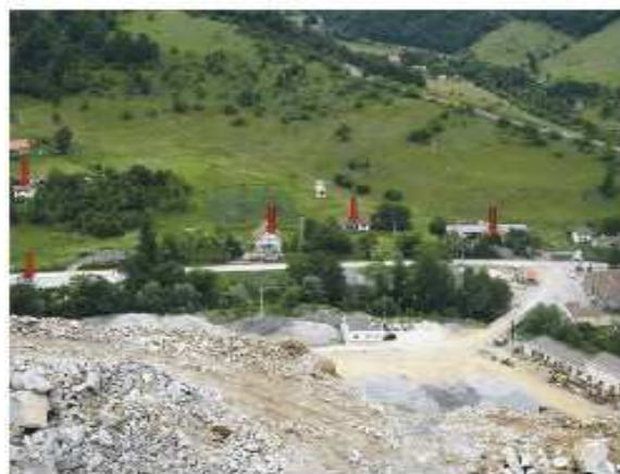
Fig. 1. Position of the objects damaged by the flyrocks
