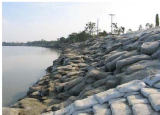
Fig. 5: Sandbags on embankment slope
