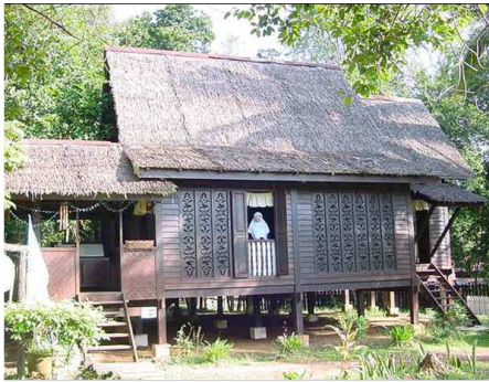
Fig. 2: Traditional Penang Malay house with Rumah ibu (middle), anjung (left) and gajah menyusu (right) additions
