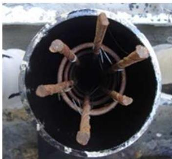
Fig. 1: Reinforcement cage in formwork
