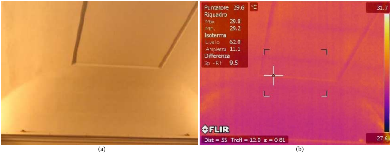
Fig. 5: Room n. 2. (a) view of the intrados of the vault (b) thermographic image showing the timber structure
