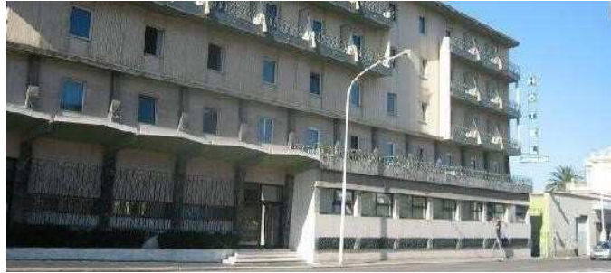
Fig. 2: Front view of the hotel
