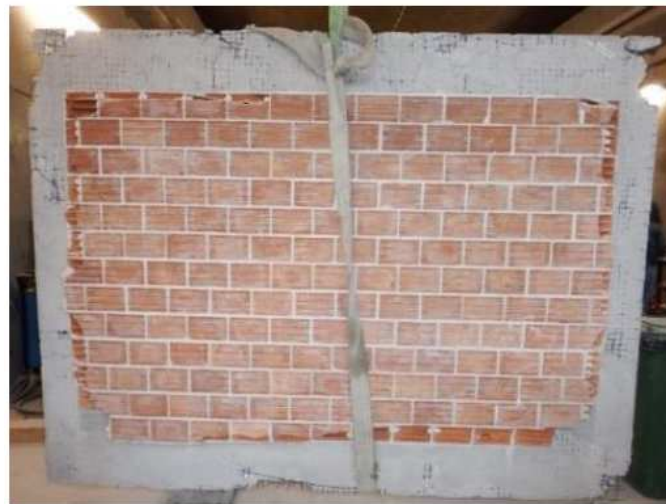
Fig. 14: View of the crushing of bricks of the infill after removing some parts of the retrofitting layer in specimen SIF(DTRM)-I
