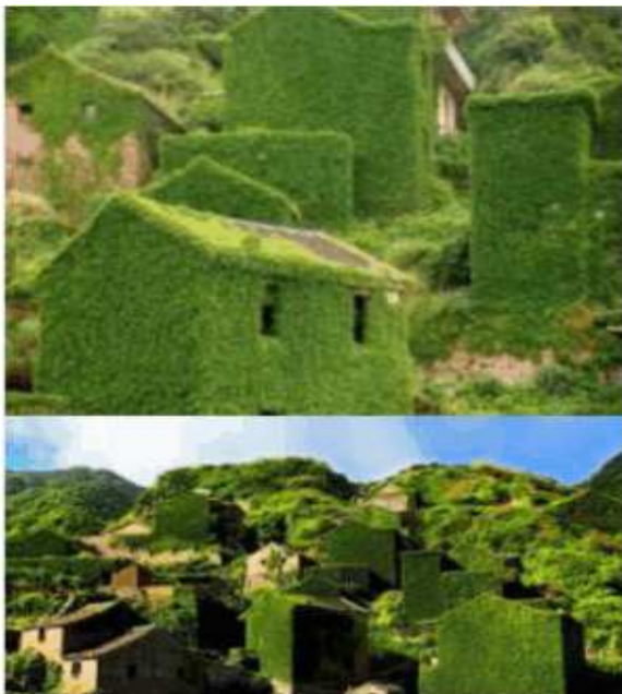
Fig. 38. "A large green" which invaded the abandoned buildings in the island of Gouqi Source: http://www.amusingplanet.com/2015/06/an-abandonedfishing-village-on-gouqi.html
