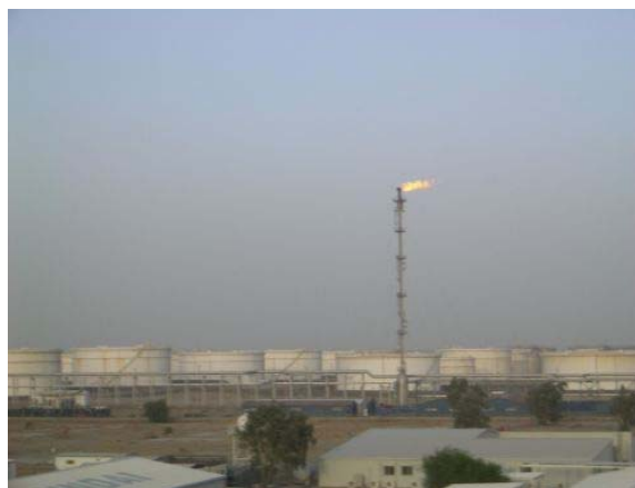
Fig. 1: Oil tank farms in Kuwait
