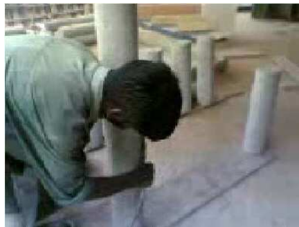
Fig. 1c: Cleaning with compressed air
