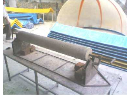
Fig. 1d: Column ready for wrapping
