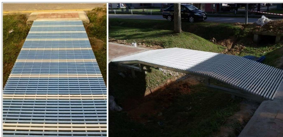
Fig. 3. Pultruded glass fibre composites grating for pedestrian bridge. (Courtesy of Rasidin Senawi, Innovative PultrusionSdn. Bhd. Seremban, Malaysia)
